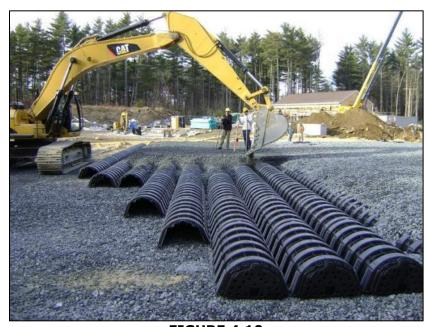
**FIGURE 4.10**Seepage Bed with Infiltration Chambers Under Construction
