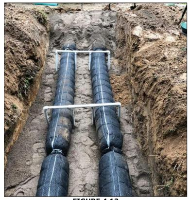
**FIGURE 4.13**Gravelless Geotextile Sand Filter Trench System (by Infiltrator)
