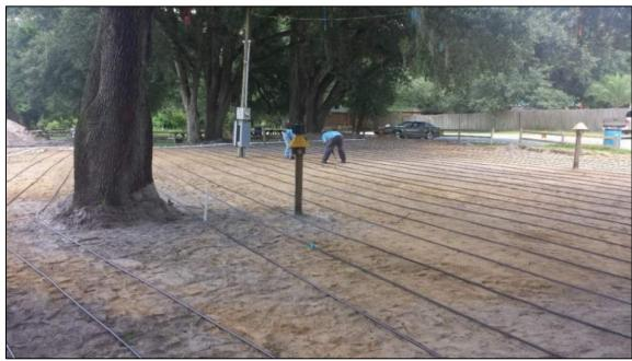
**FIGURE 4.11**Drip Dispersal System Before Backfill
