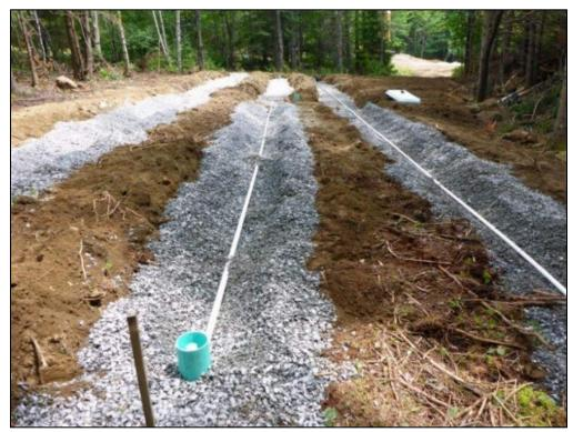
**FIGURE 4.9** Typical Trench Absorption Field Under Construction
